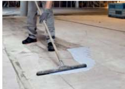
Floor coating: the prepared, oil-free floor surface must be evenly primed with PCI Gbsgrund® 404 before a cementitious floor levelling compound is used.
