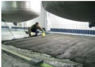
The PCI Novaman ® product family includes fast-setting screeds for mixing on site and ready-mixed mortars.
