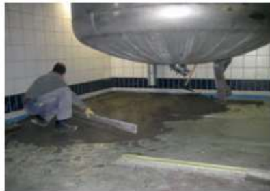
Screed laying with fast-setting PCI Novaman ® M1 plus.
