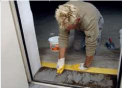
The ready-to-use PCI Aposar® is applied to the dry, primed floor ...
