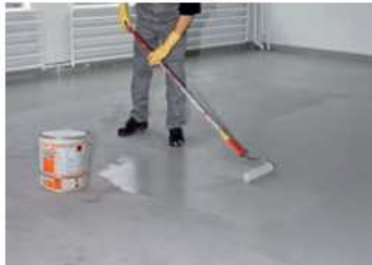
When it has cured and dried, the coating may be sealed using PCI Apoker® W. The epoxy resin sealing compound PCI Apoker® W must be mixed evenly and then evenly applied with cross-wise motion using a roller.
