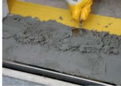
... pressed into place and compacted using a trowel...
