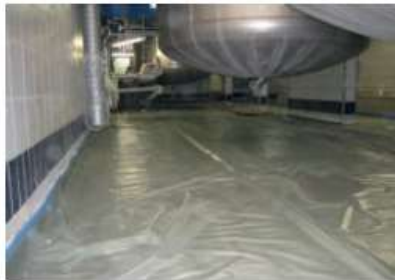
Placing an insulating layer on the unsealed concrete.
