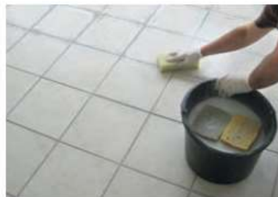
Tiling and grouting with acid-resistant PCI Durapox ® NT plus.
